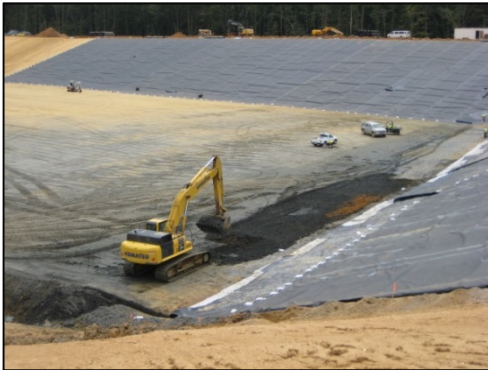
Installation of the Liner System
